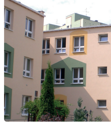
Rehabilitation Clinic of Zgorzelec
